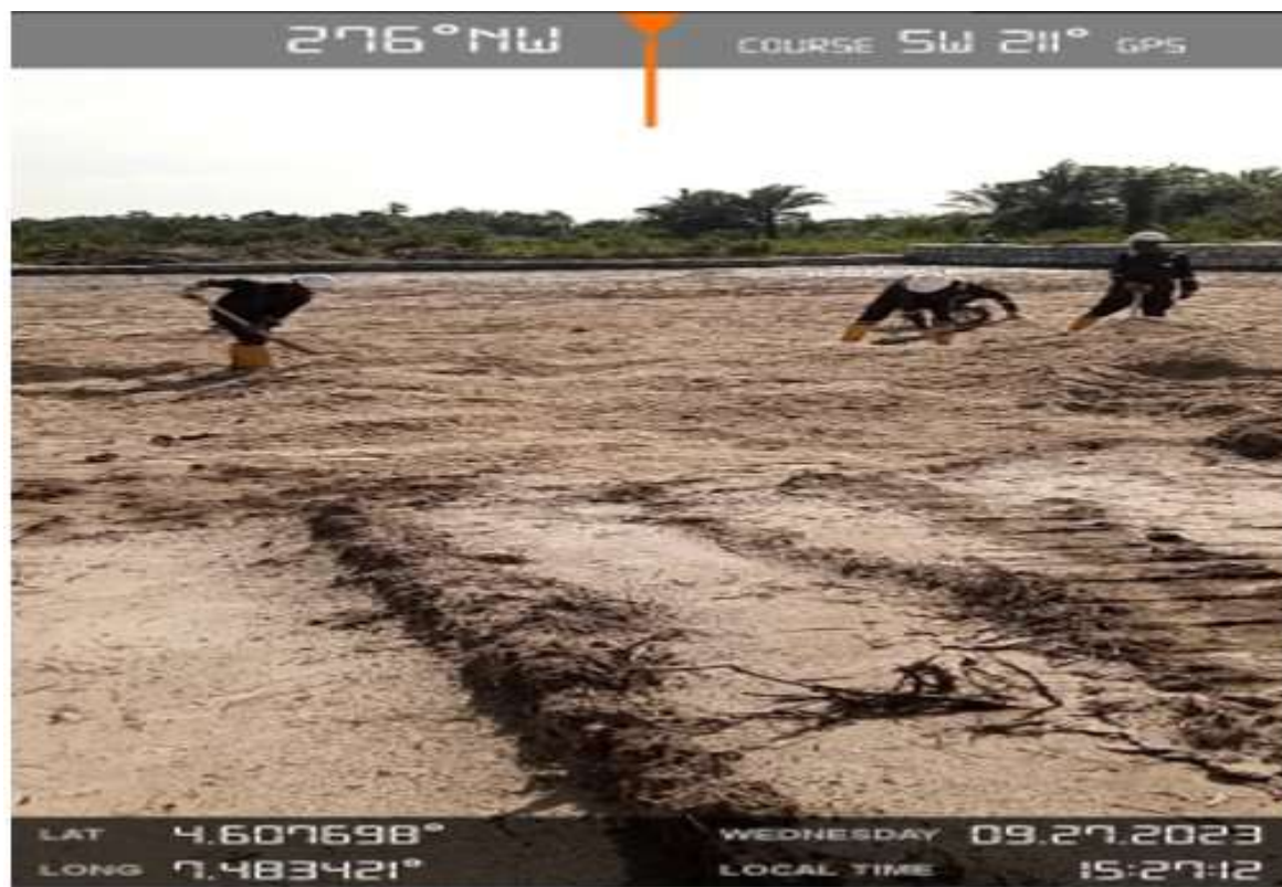
Plate 2: Levelling of the Biocell
