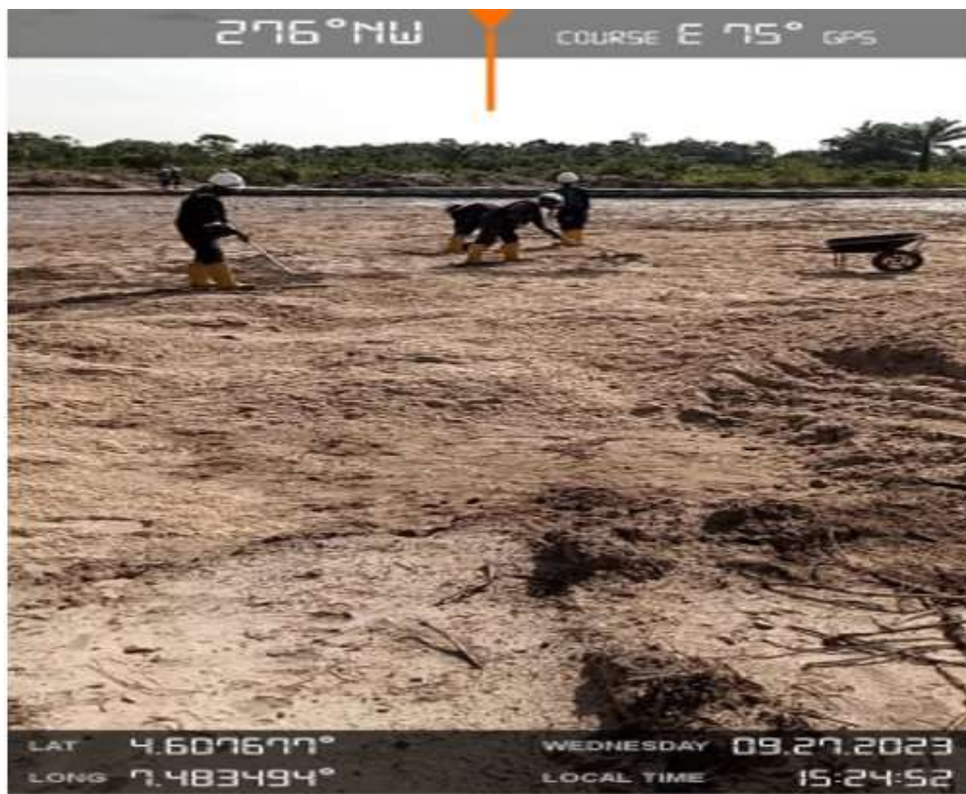
Plate 4: Surface Preparation/Raking of the Biocell
