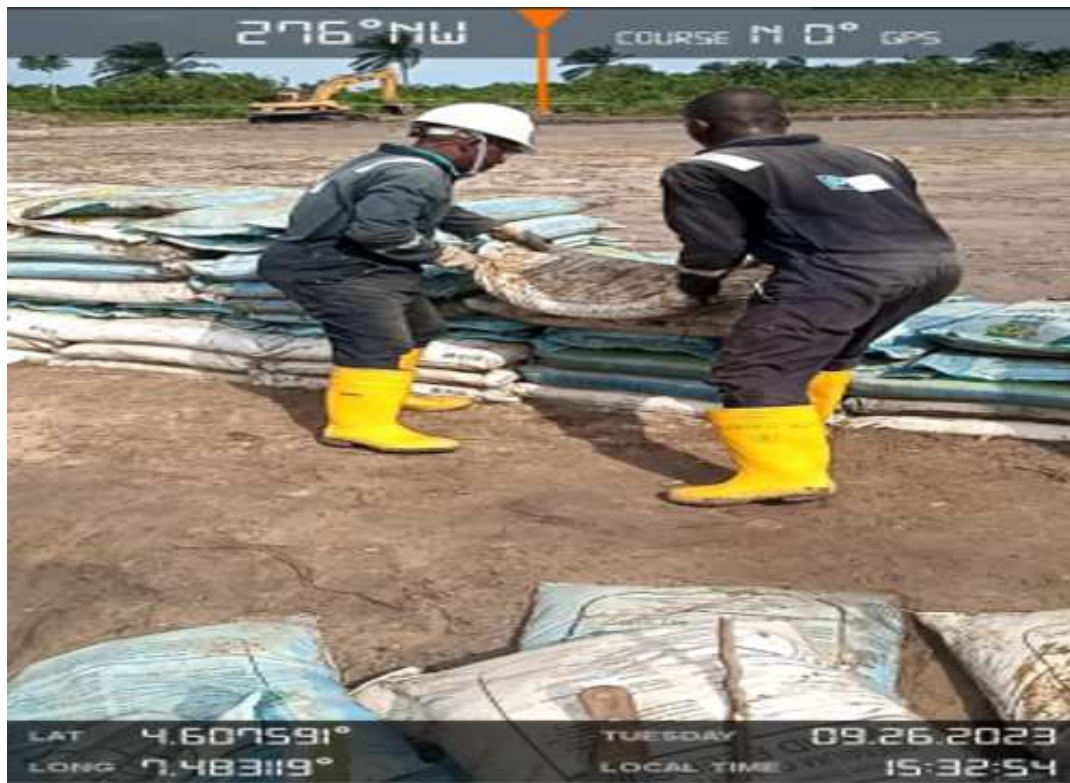
Plate 3: Stacking of Sandbags
